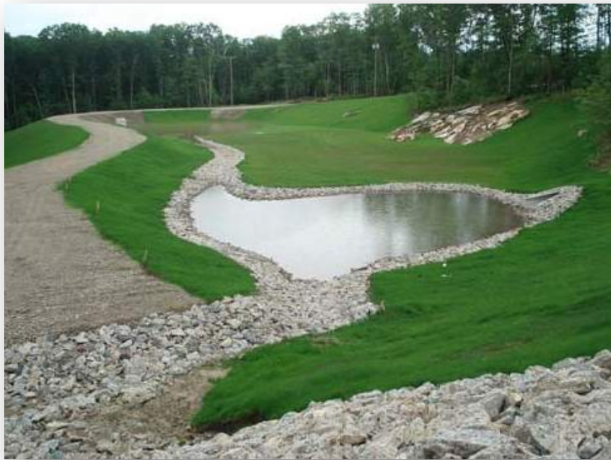
Photo: Example of a linear string of BMPs, including temporary storage.
