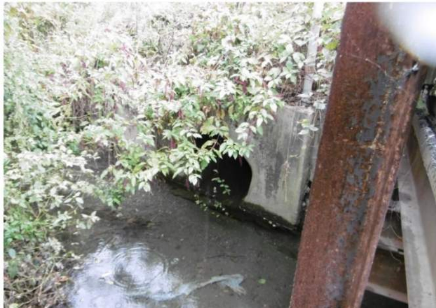
Photo: View from the bridge at outfall #6. Image shows sediment accumulated along channel floor
