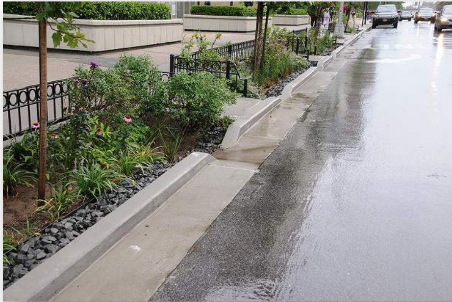
Photo: Example of street bioswale area. Curb cuts channel runoff to the vegetated areas for filtering out sediment and pollutants.
